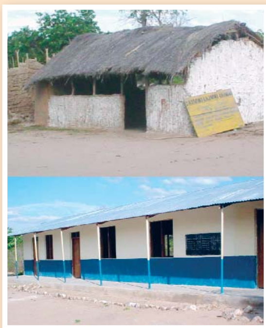
Figure 13: One of the ACCESS Centers before and after rehabilitation
