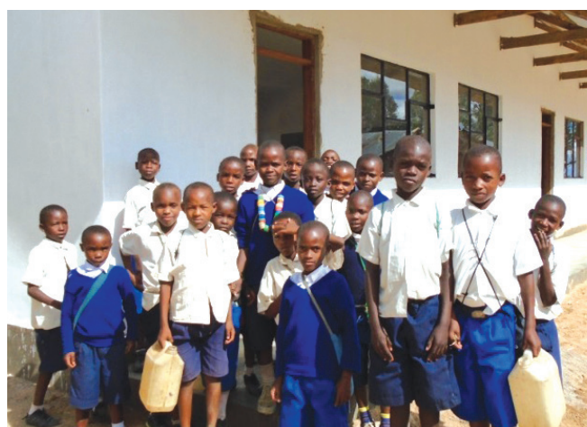
School block in Mrama Village (child sponsorship area), Chamwino district which is constructed in response to community demand, The community played a leadership role in mobilization and demand the local government support
