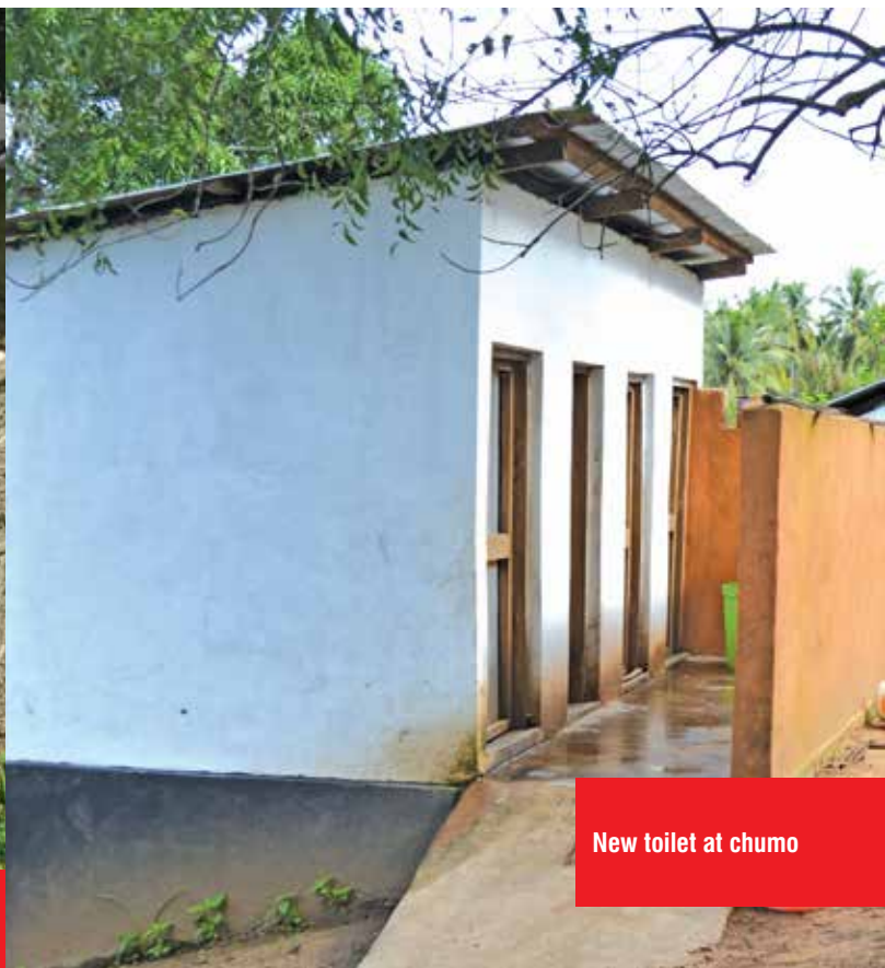
Toilets at chumo last year
