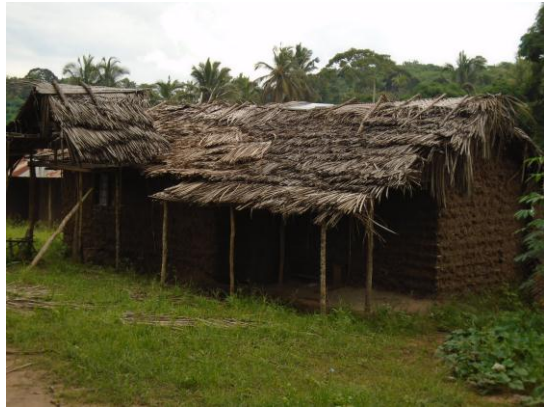
One of the teachers' house built using local materials by community members despite the fact that community around has modern houses at Kibata primary school
