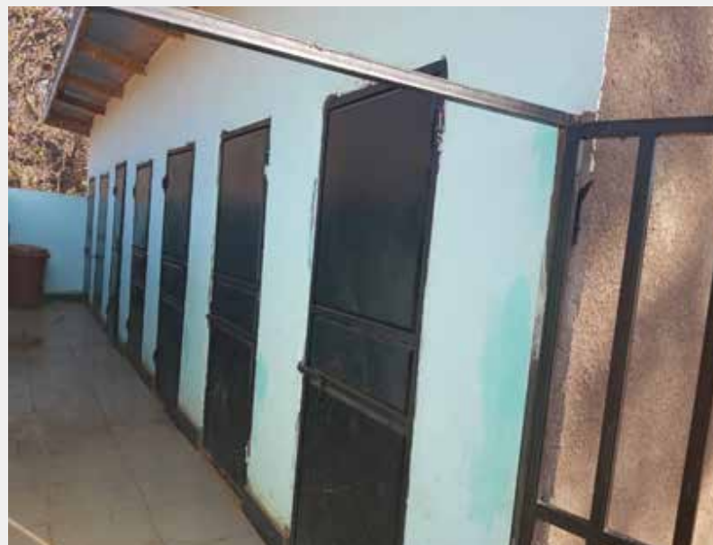
Newly constructed toilets in Nchoya Primary School
